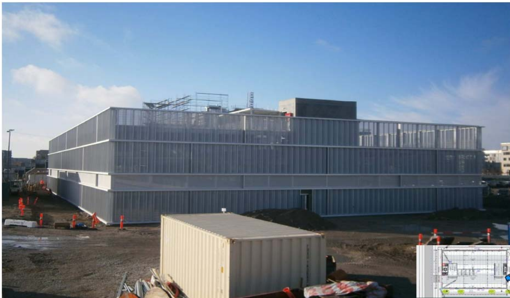
B.2/ PICTURE NO. 2 - VIEW FROM THE EAST – GL 23
